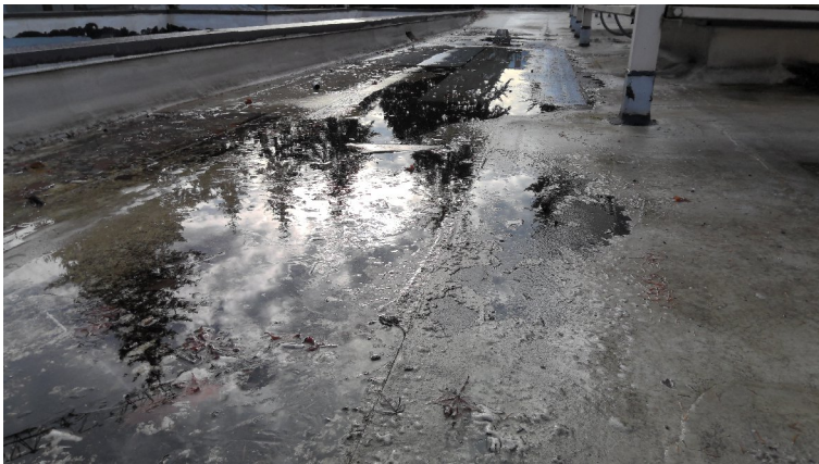
End-of-Life Roofing (Fire Station 11)
