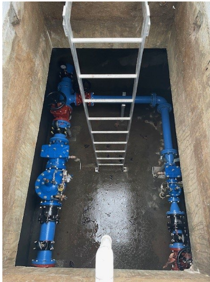
View looking down into PRV Vault
