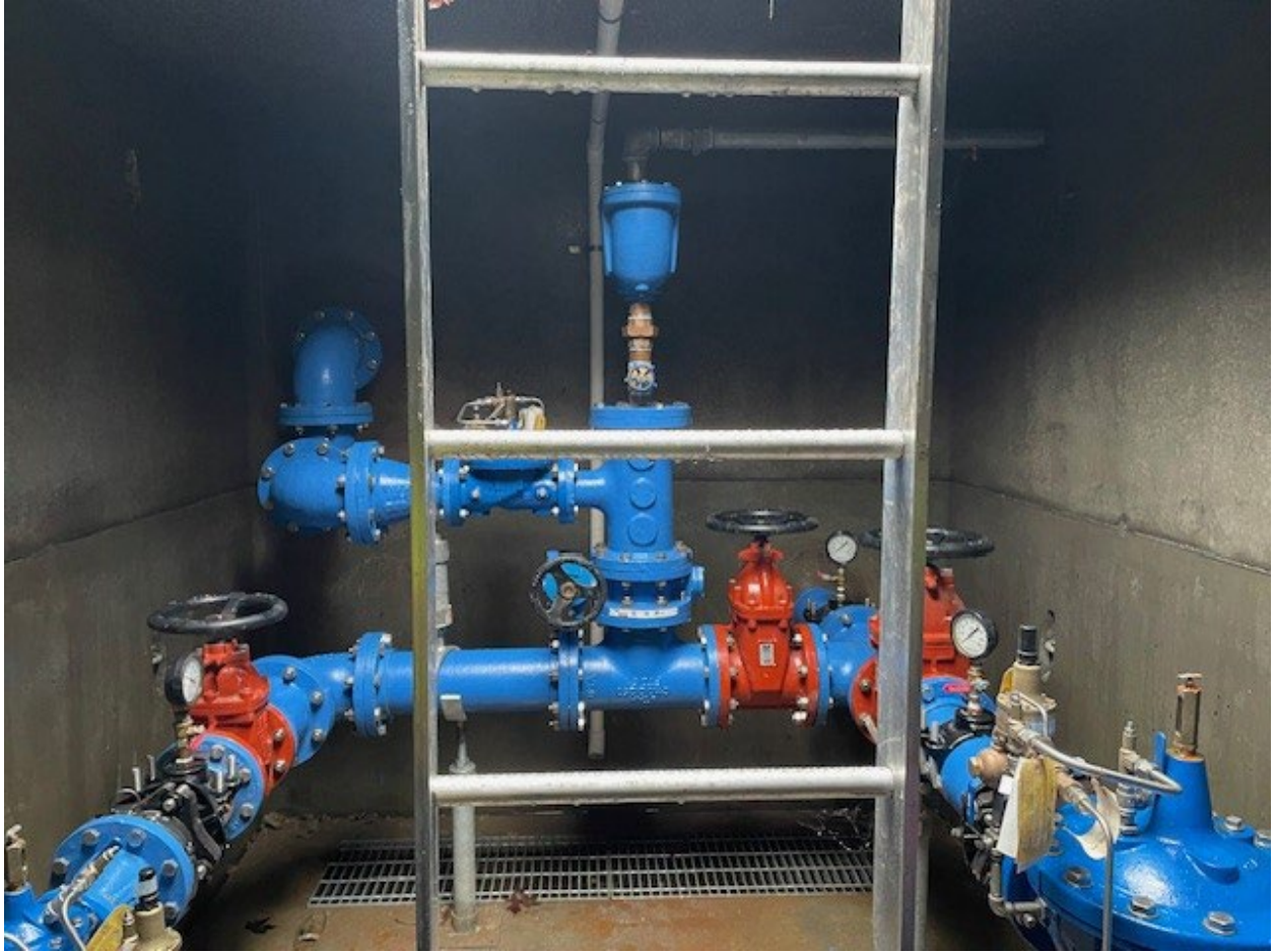
View inside PRV Vault
