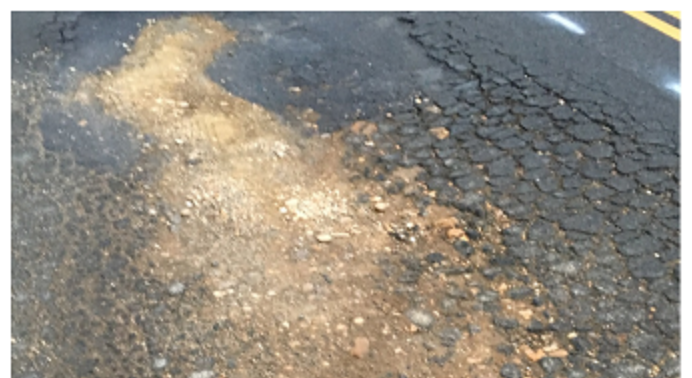
Pavement Condition 0 - 10 (Failed)
