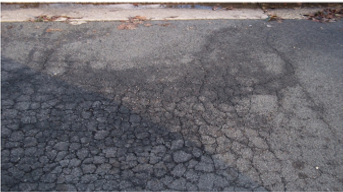
Pavement Condition 11 - 40 (Very Poor/Serious)
