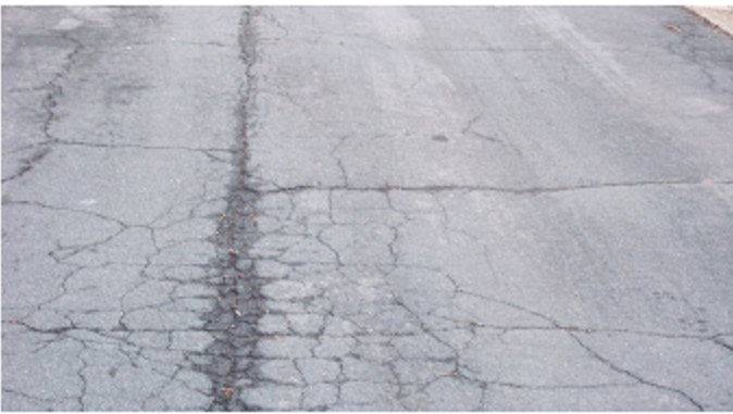
Pavement Condition 41 - 55 (Poor)
