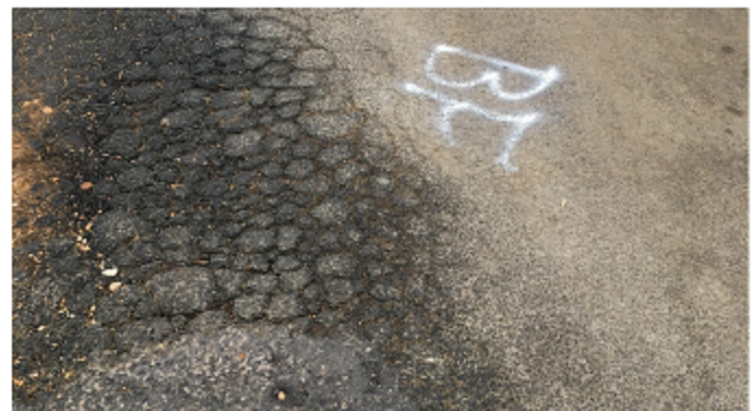
Pavement Condition 0 - 10 (Failed)
