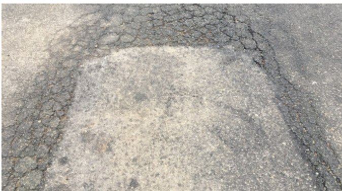
Pavement Condition 0 - 10 (Failed)
