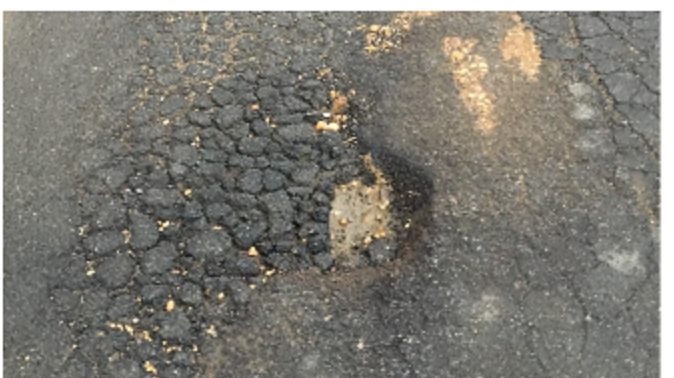
Pavement Condition 0 - 10 (Failed)
