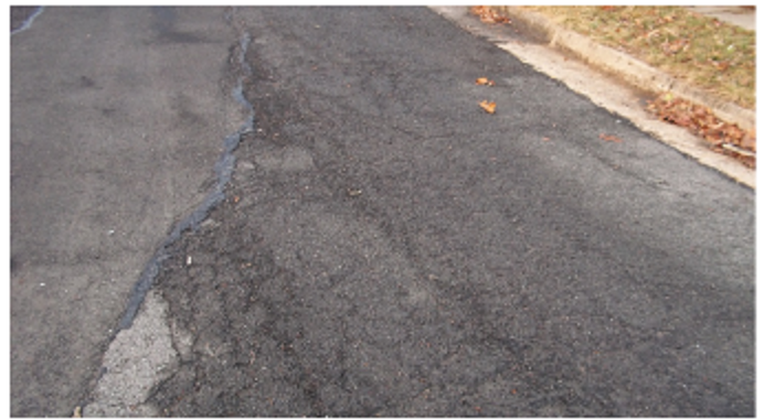
Pavement Condition 41 - 55 (Poor)
