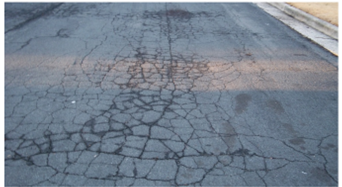
Pavement Condition 11 - 40 (Very Poor/Serious)
