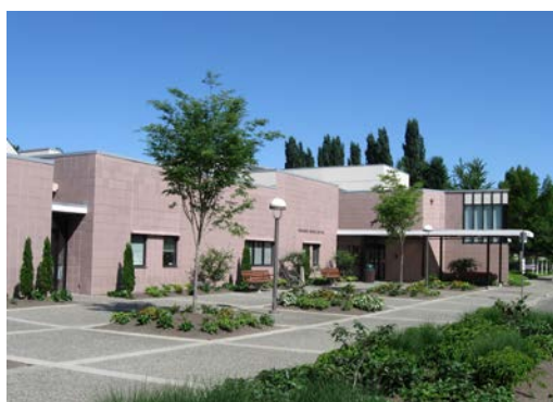
Photo: Existing Redmond Senior Center Courtesy: City of Redmond
