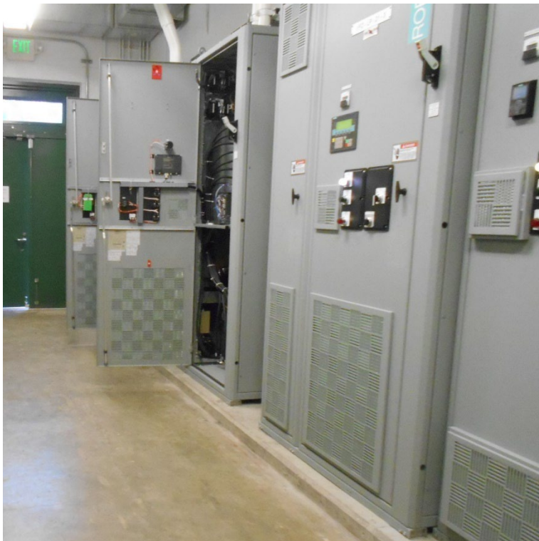
Trilogy Pump Station VFDs
