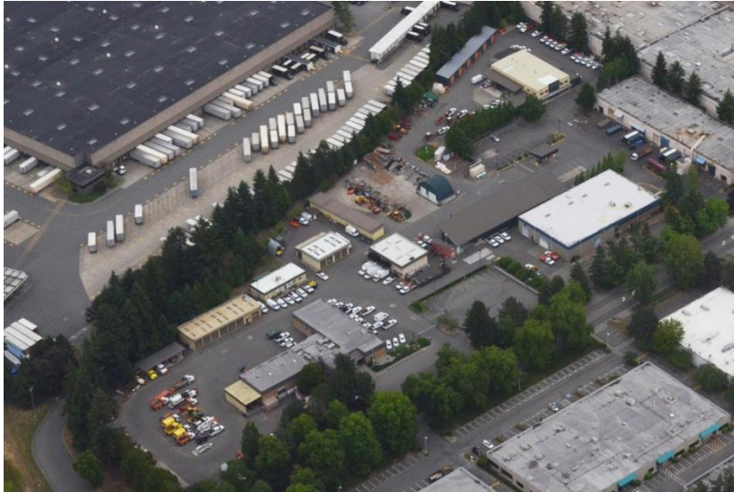
Aerial view of the Maintenance & Operations Center
