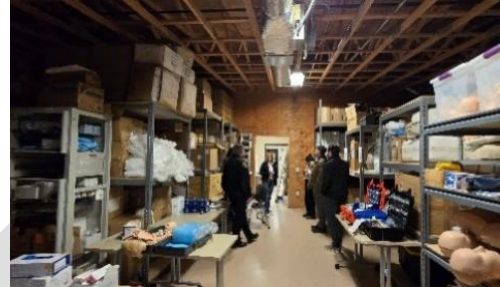
Unfinished space at Fire Station 17
