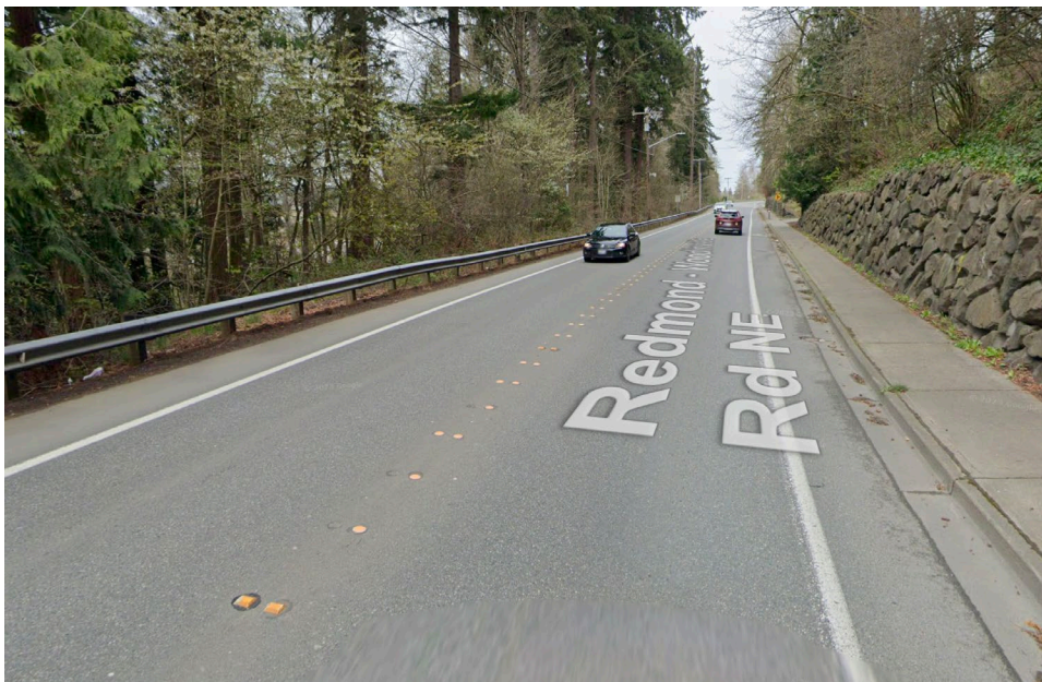
Figure 1: View north along Redmond-Woodinville Road Showing Standard Bike Lanes and an Unbuffered Sidewalk (source: Google, 2023)
