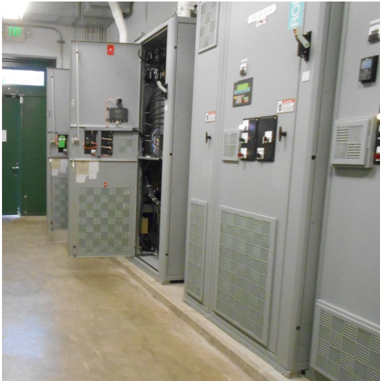
Trilogy Pump Station VFDs
