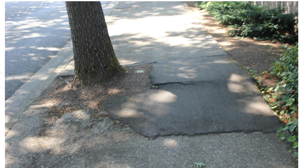
Future Path Project, east of 163 rd Ave.: damaged sidewalk repair
