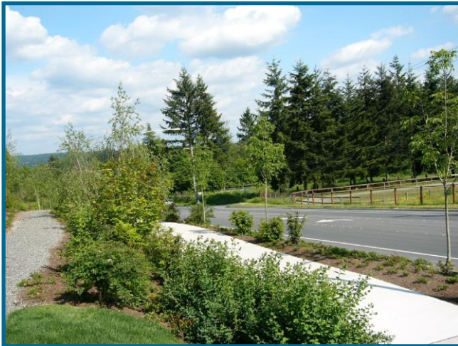
Improvements along NE 116th St.
