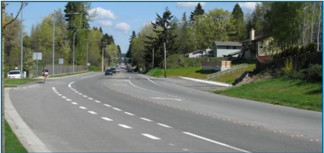
Improvements along Red-Wood Road
