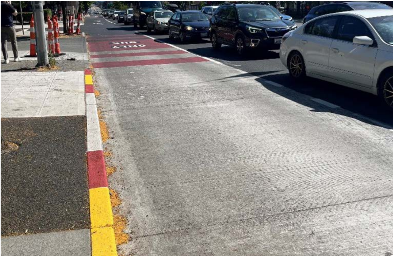
FIGURE 5 | CONCRETE BUS PADS REDUCE IMPACTS OF HEAVY BUSES ON PAVEMENT
