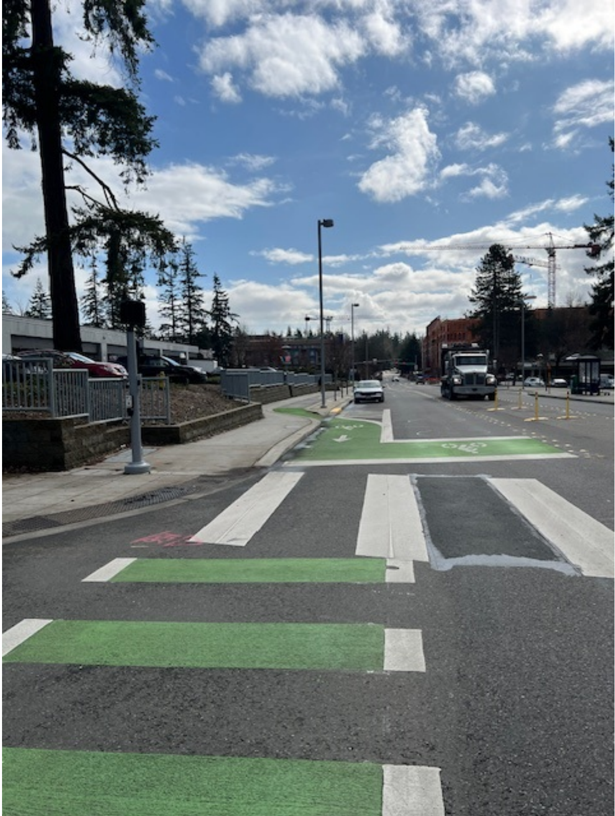
Northbound Lane at NE Hopper St
