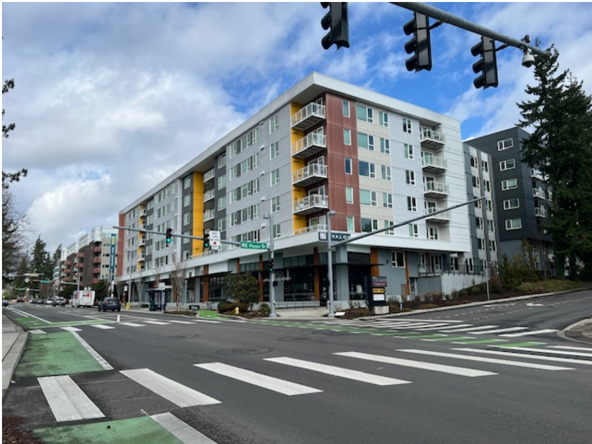
Intersection at Hopper St
