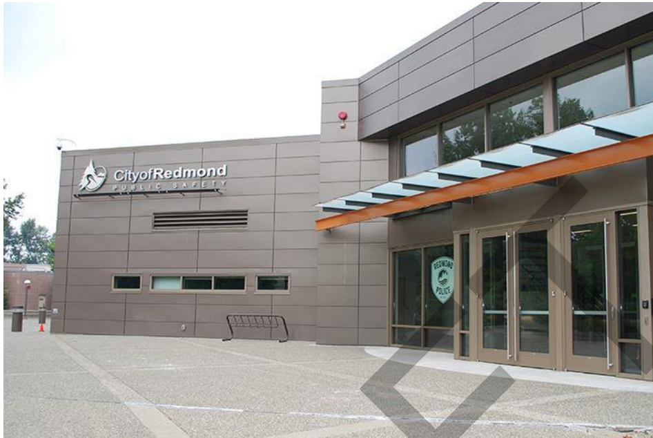
FIGURE 6: REDMOND PUBLIC SAFETY BUILDING
