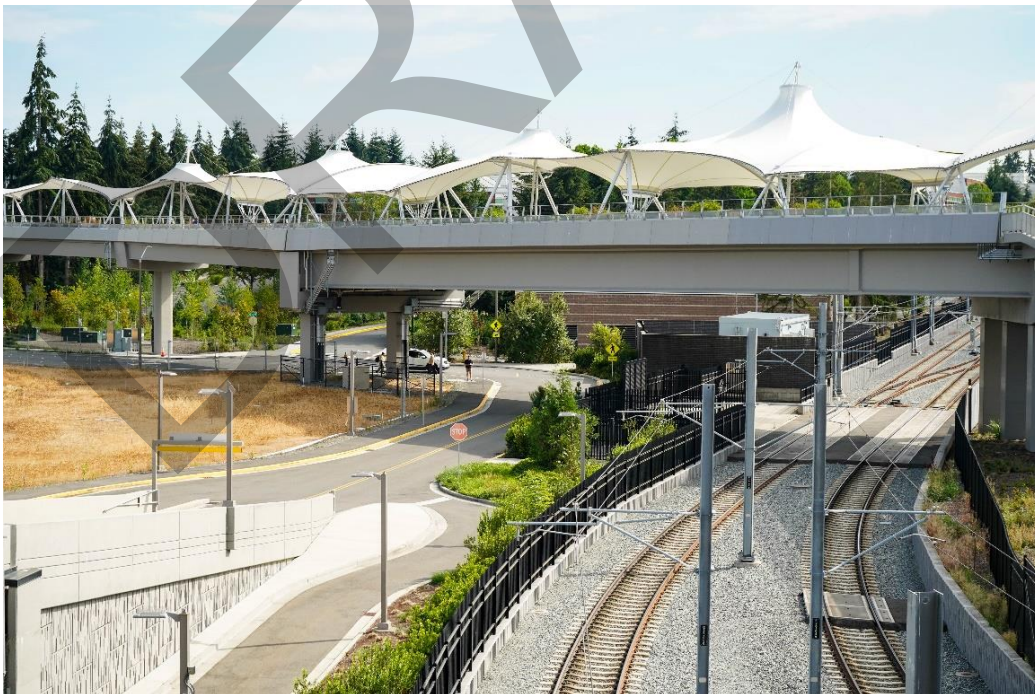
FIGURE 4: RTS PEDESTRIAN BRIDGE
