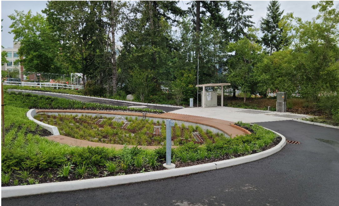
Pump equipment in background with Filtterra Bioscape in foreground
