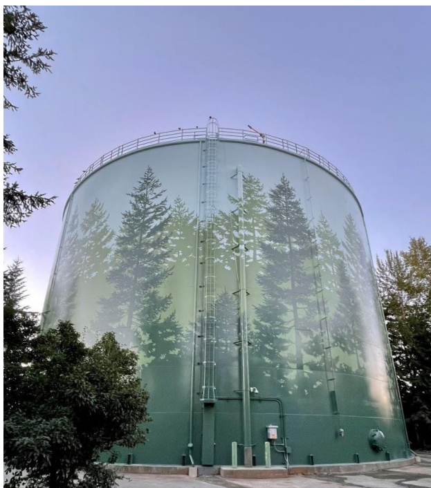
FIGURE 13: SE REDMOND WATER STORAGE TANK
