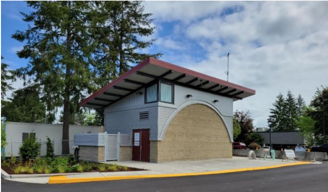
FIGURE 14: LIFT STATION 13 (MARYMOOR)
