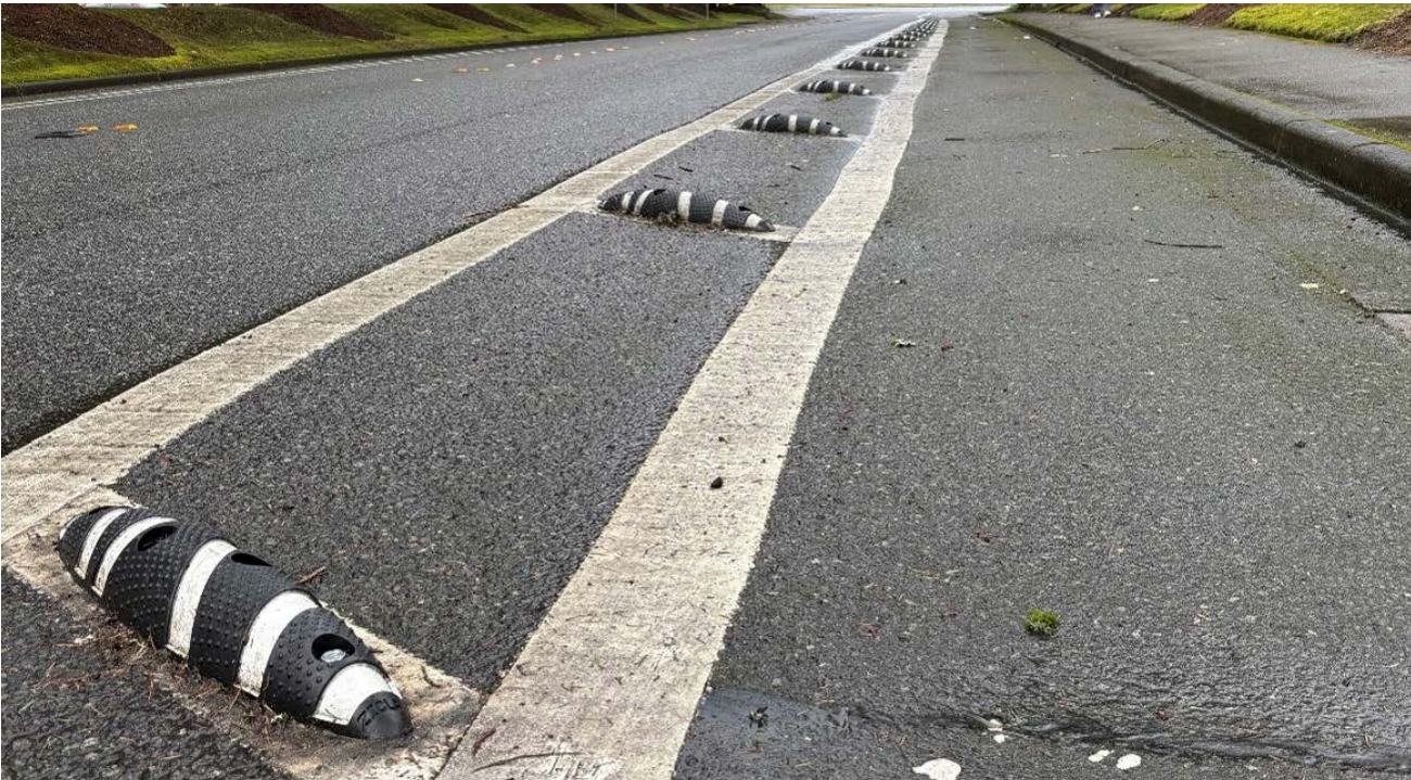
FIGURE 7 | QUICK BUILD MATERIALS SUCH AS THESE “ARMADILLOS” ON THE 150TH AVE NE BIKE LANE CAN BE USED TO ROLL OUT NEW HIGHER COMFORT BIKEWAYS MORE RAPIDLY
