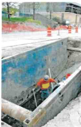
An example of open-trench construction.
