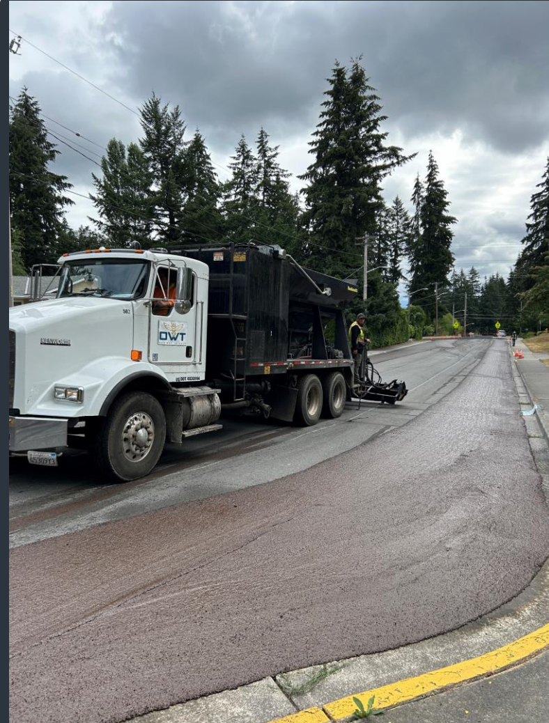
2024 Residential Preventative Maintenance Slurry Seal
