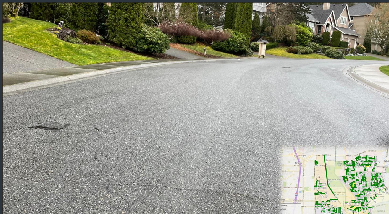
North Redmond 179 th Court Residential Street
