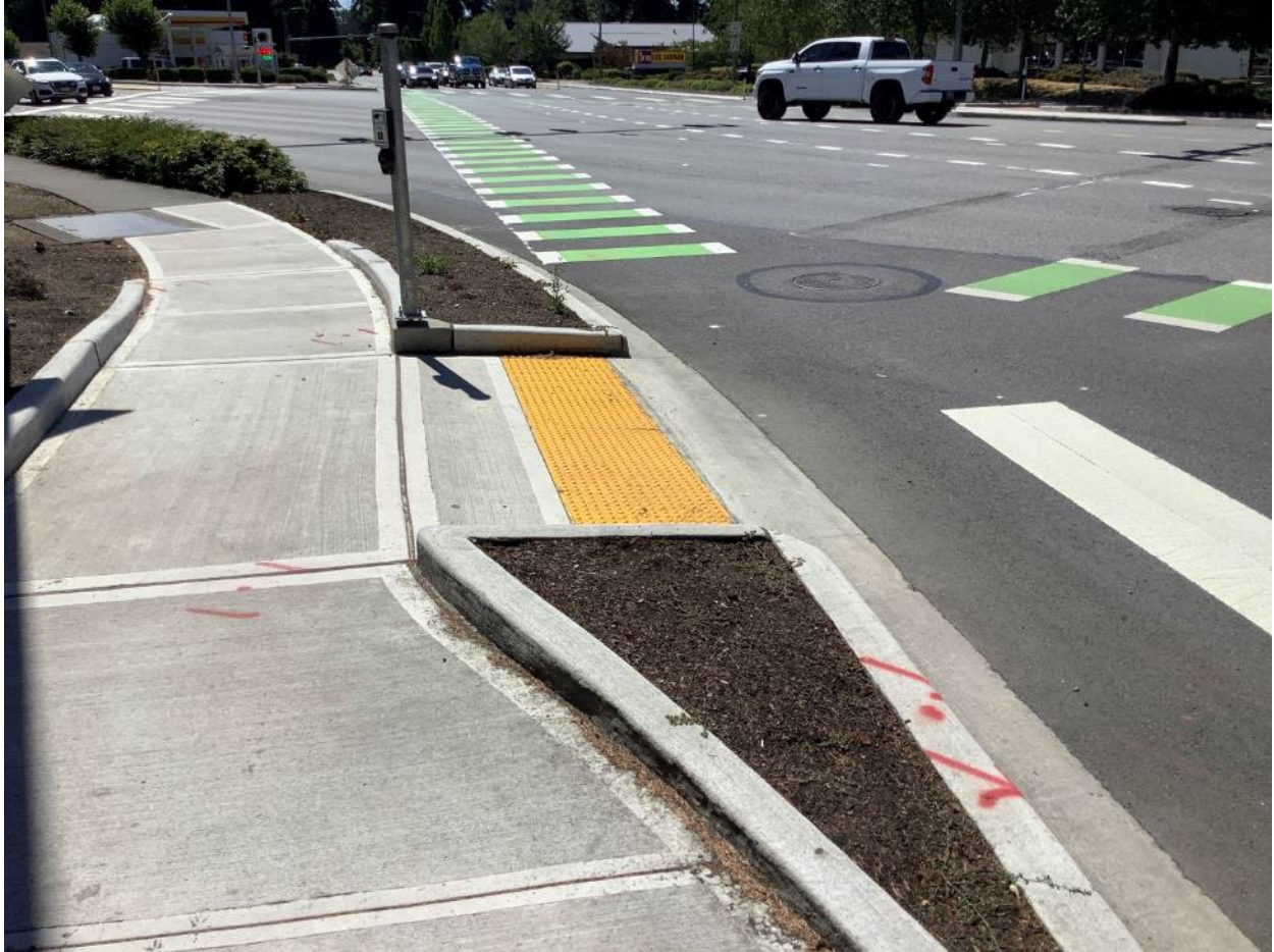
ADA compliant curb ramp
