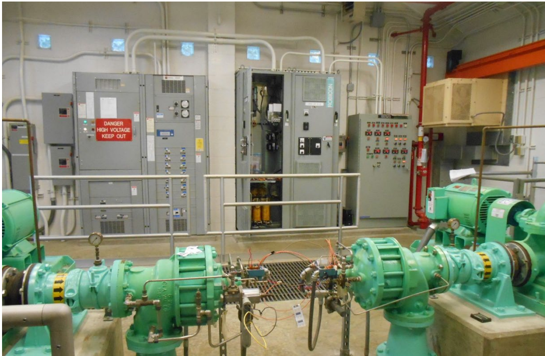
Novelty Hill Operations Center VFDs (the two tall units on the right)
