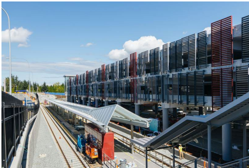
Sound Transit rendering of Redmond Technology Station light rail station in Redmond's Overlake neighborhood. Source(s): soundtransit.org
