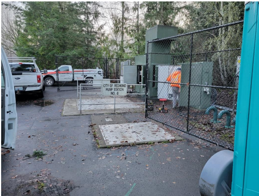
Wastewater Lift Station 8 during construction
