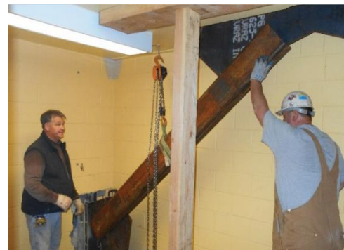
Seismic upgrade work at the Public Safety Building
