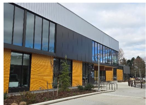
The Redmond Senior & Community Center is an all-electric building
