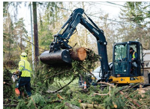
City crews clear debris from the 2024 “bomb cyclone” weather event
