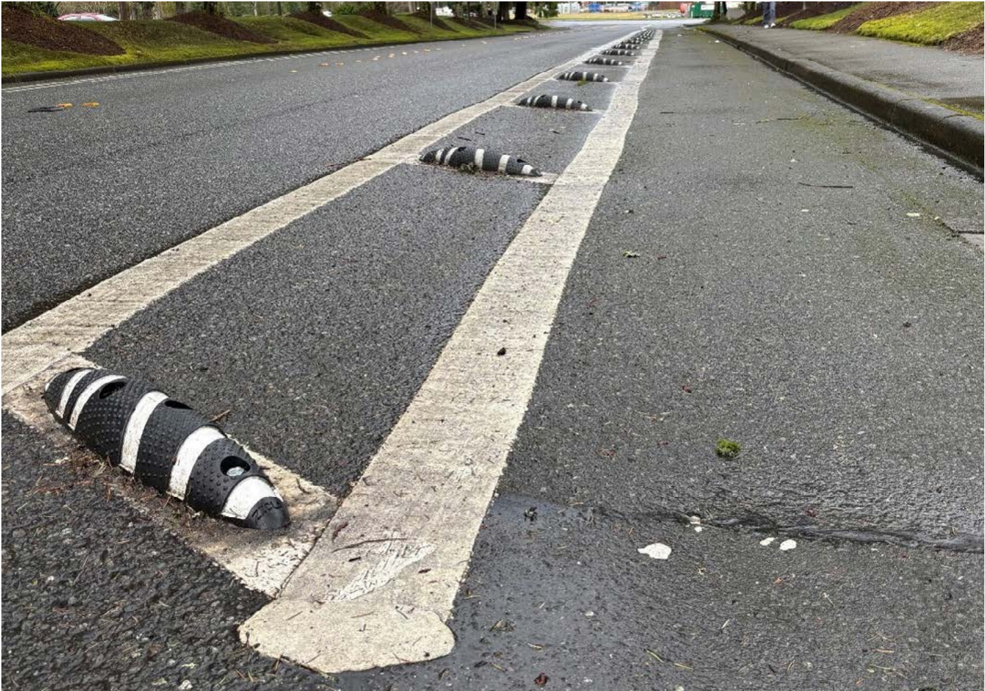
FIGURE 7 | QUICK BUILD MATERIALS SUCH AS THESE “ARMADILLOS” ON THE 150TH AVE NE BIKE LANE CAN BE USED TO ROLL OUT NEW HIGHER COMFORT BIKEWAYS MORE RAPIDLY
