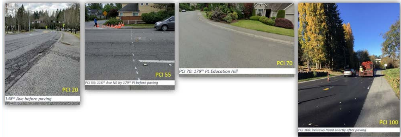
FIGURE 1 | VISUAL EXAMPLES OF PAVEMENT CONDITION
