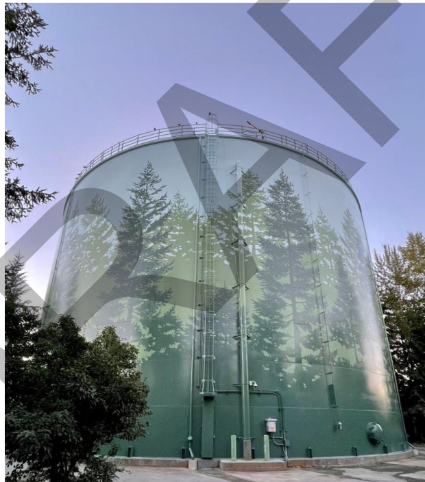
FIGURE 13: SE REDMOND WATER STORAGE TANK
