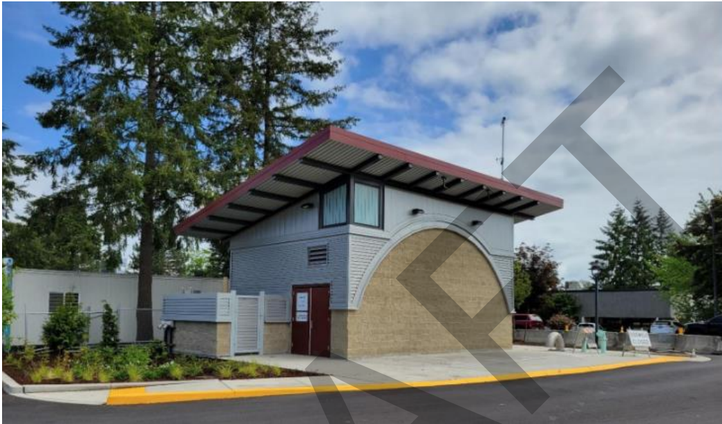
FIGURE 14: LIFT STATION 13 (MARYMOOR)
