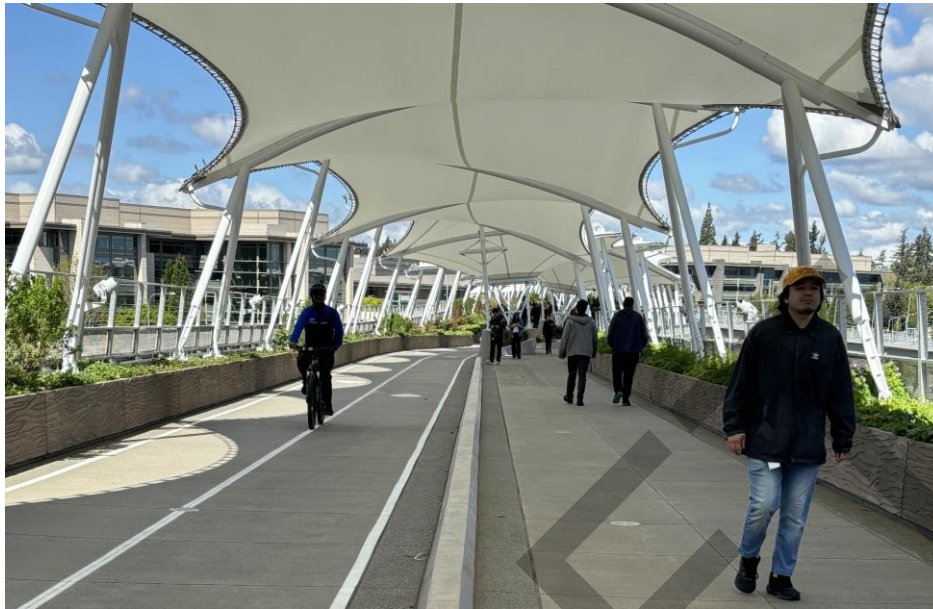
FIGURE 11: RTS PEDESTRIAN BRIDGE
