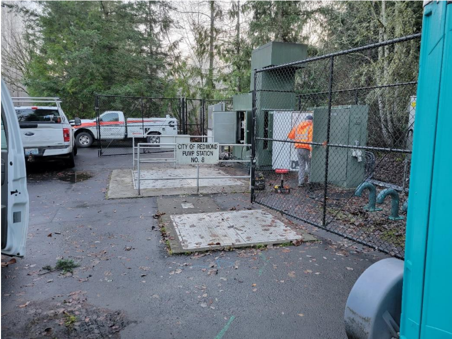
Wastewater Lift Station 8 during construction
