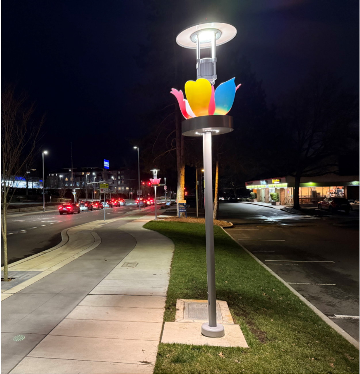
Artistic Lighting installed along 152 nd Ave NE
