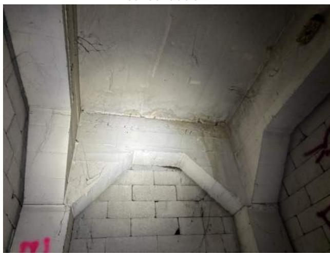
Image VI.18 Hose Tower concrete frame
