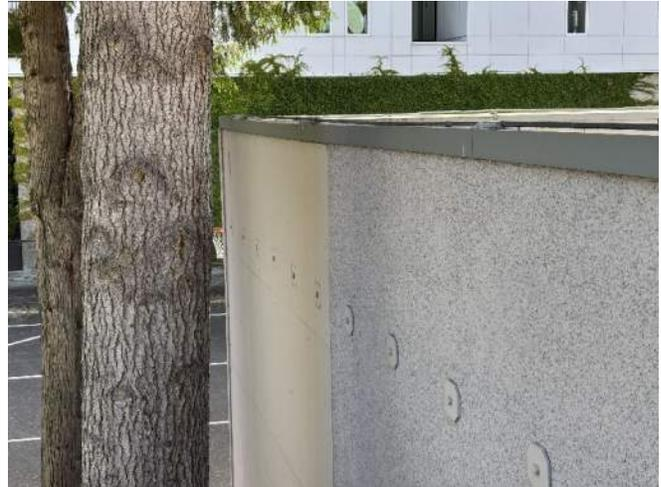
*Image VI.8 Exterior roof to wall anchorage*
