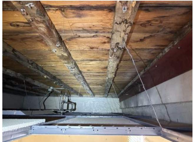
*Image VI.14 Water-damaged roof decking in couch room*
