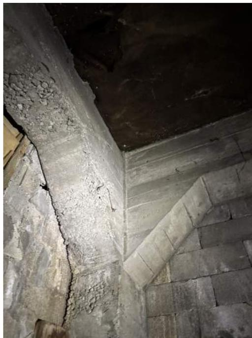
Image VI.16 Hose Tower concrete frame with poor consolidation
