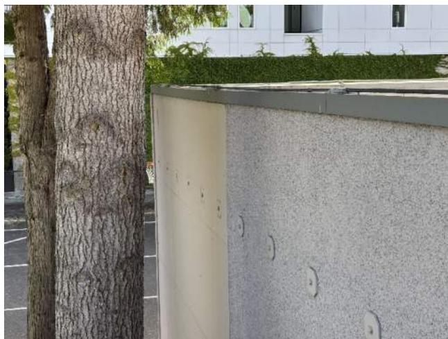
*Image VI.8 Exterior roof to wall anchorage*
