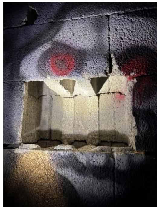
Image VI.22 Broken CMU block in Hose Tower wall
