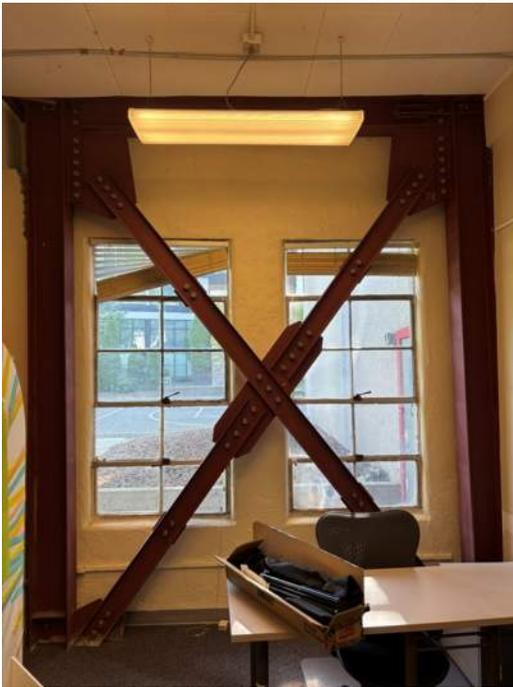
Image VI.3 Braced Frame on GL 5
