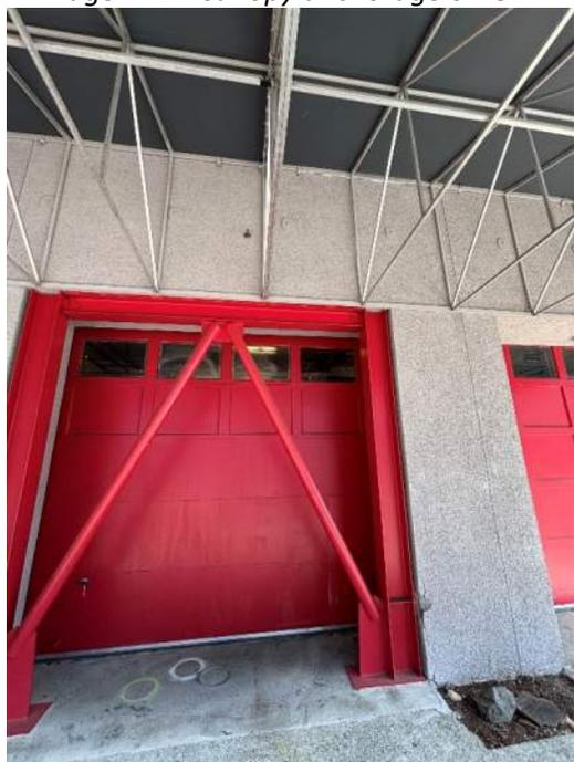
*Image VI.13 Braced Frame on GL F*
