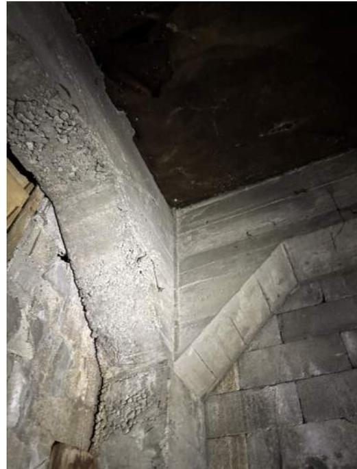
Image VI.16 Hose Tower concrete frame with poor consolidation
