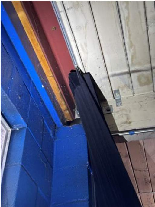
Image VI.5 Roof framing at pilaster in Showroom
