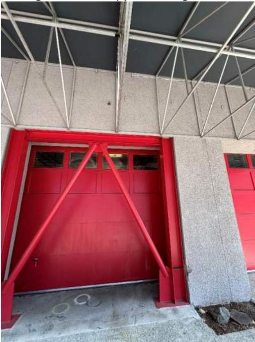
*Image VI.13 Braced Frame on GL F*
