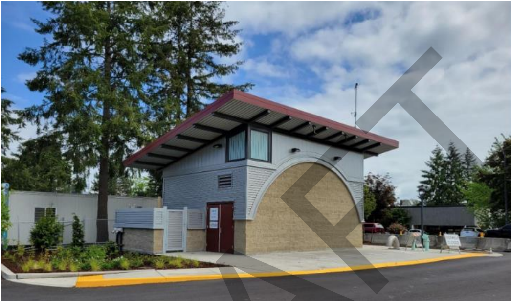
FIGURE 14: LIFT STATION 13 (MARYMOOR)
