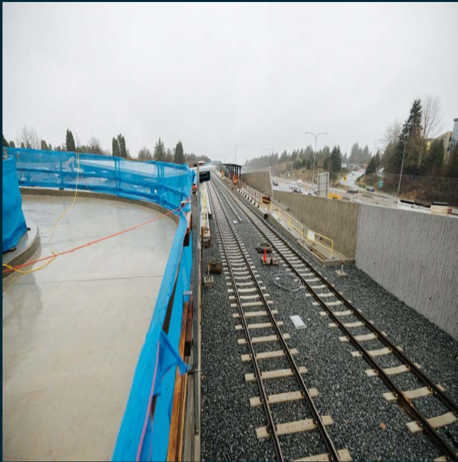
OVS Bridge and Tracks looking southwest
