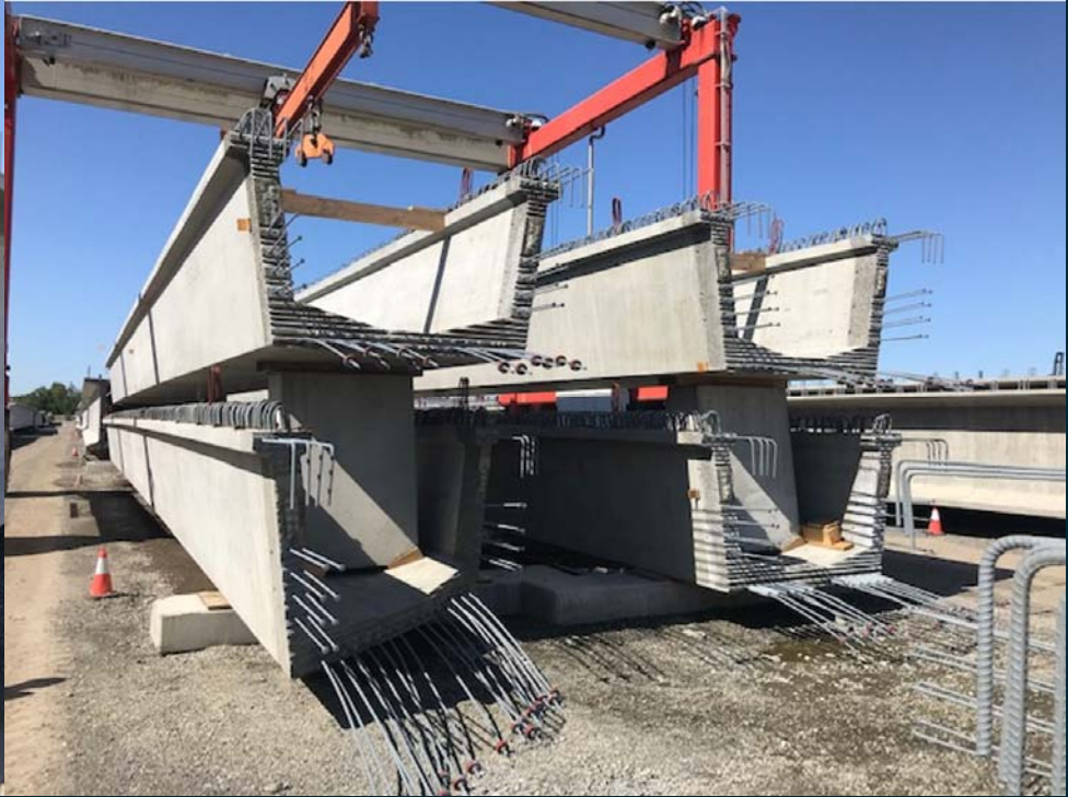
"Tub" girders ready to ship to the site 5' high, 8' wide (top), 105' long, 80 tons
