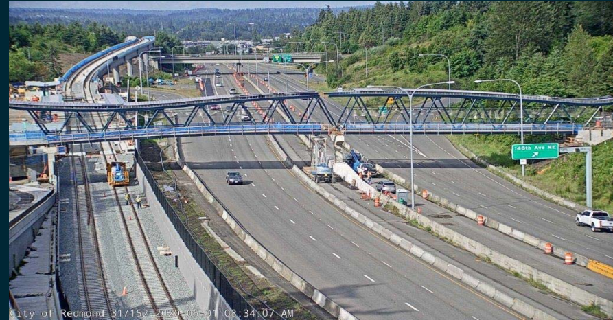
OVS Ped-Bike Bridge truss setting is complete over SR520
