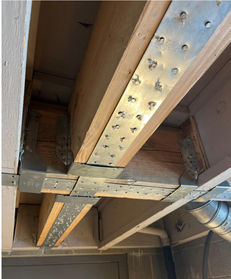
Example of seismic bracing in ceiling
