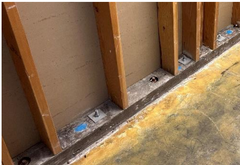
Example of seismic anchor bolts at foundation
