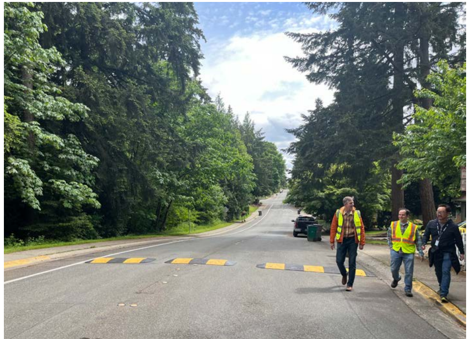
Typical residential street observed during City RSA
