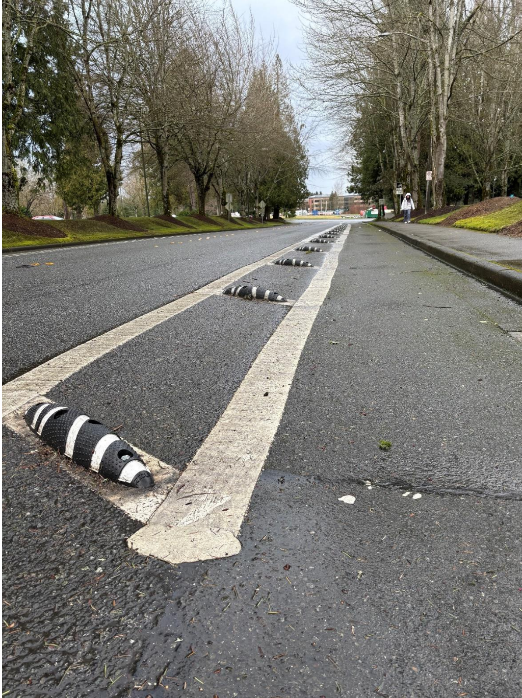
FIGURE 7: QUICK BUILD MATERIALS SUCH AS THESE "ARMADILLOS" ON THE 150 TH AVE NE BIKE LANE CAN BE USED TO ROLL OUT NEW HIGHER COMFORT BIKEWAYS MORE RAPIDLY (IMAGE CREDIT: CITY OF REDMOND)
