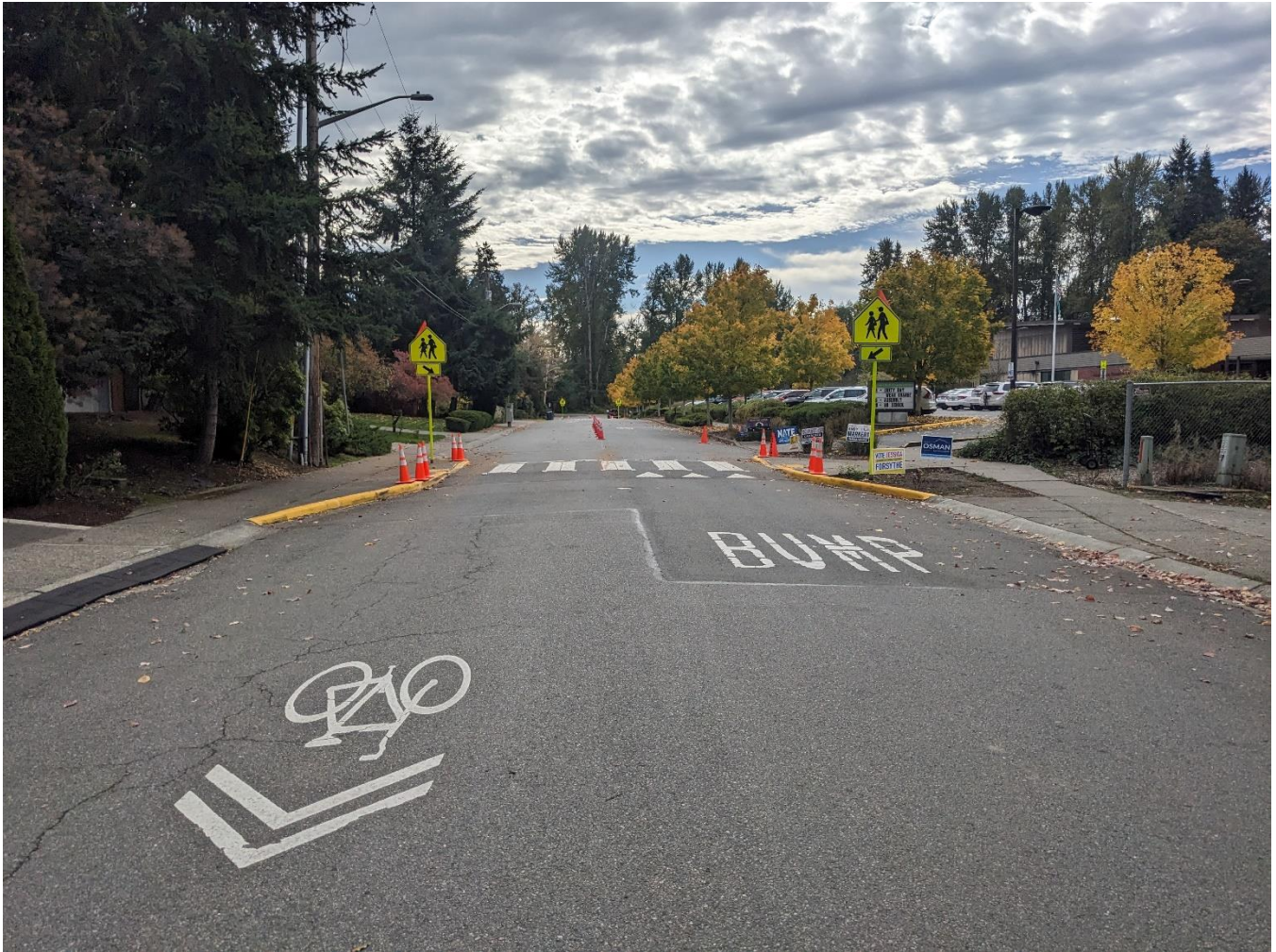
FIGURE 11: TRAFFIC CALMED BICYCLE BOULEVARDS SUCH AS THIS ONE ON 152 ND AVENUE NE IN REDMOND PROVIDE IMPORTANT CONNECTIONS BETWEEN HOMES AND NEIGHBORHOOD DESTINATIONS LIKE SCHOOLS AND PARKS (IMAGE CREDIT: TOOLE DESIGN)
