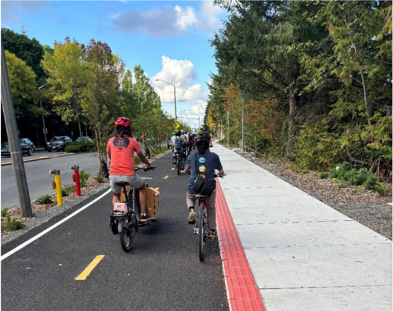
FIGURE 2: SEPARATED BIKE LANES LIKE THIS ONE ON 156 TH AVE NE PROVIDE A HIGHER LEVEL OF COMFORT AND SAFETY AND ATTRACT BICYCLISTS OF ALL AGES AND ABILITIES. (IMAGE CREDIT: CITY OF REDMOND)
