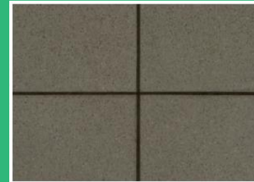
Accent Paving at Retail: Concrete Paving with Topcast Finish and Integral Color
