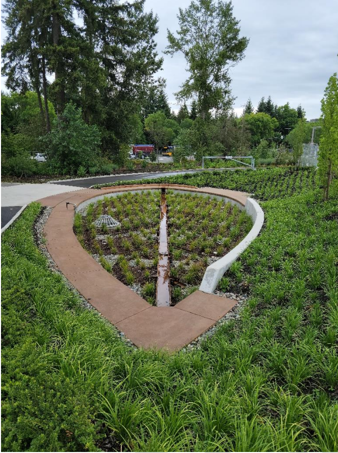
Leaf shaped Filterra bioscape
