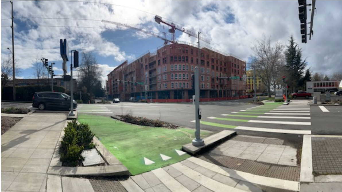
Intersection at NE 24 th St
