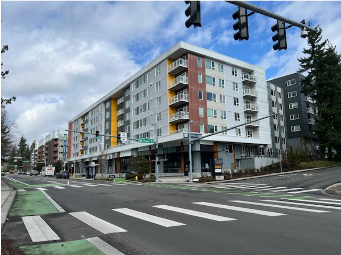
Intersection at Hopper St
