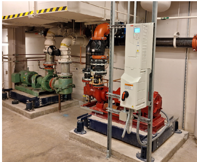
Figure 3 – Condenser Pump
