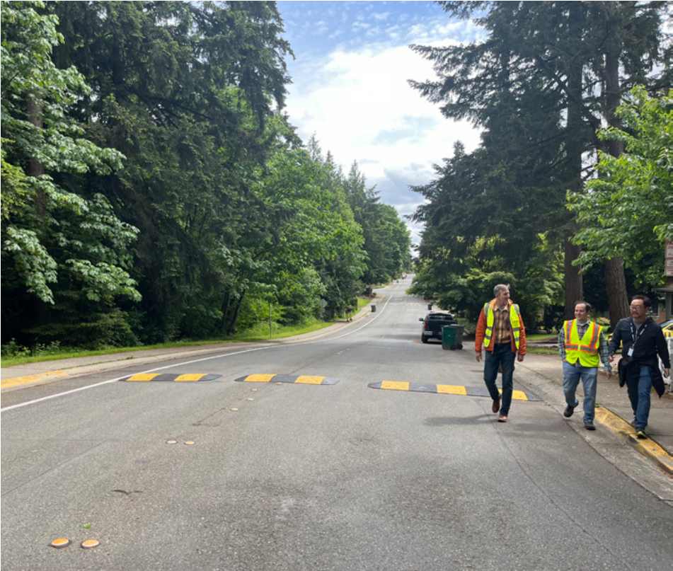
Typical residential street observed during City RSA
