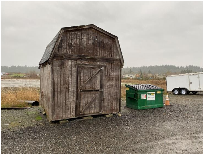
Photograph 3. Prefabricated shed on the central portion of the Property.
