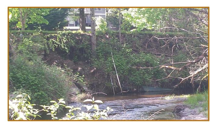
The embankment, with two stormwater outfalls and a utility pole, is being eroded by Bear Creek.
