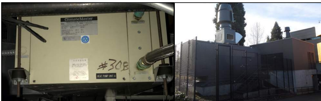
Figure 3: Typical Heat Pump and Exterior Cooling Tower
