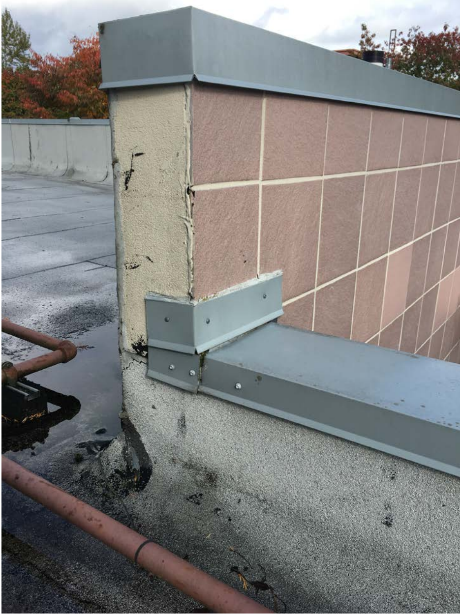
Intersection of parapets at roof showing metal surface mounted angled flashing providing protection with sealant from moisture/dry rot.
