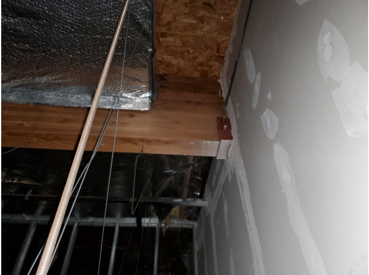
Typical observed condition of glulam roof beam
