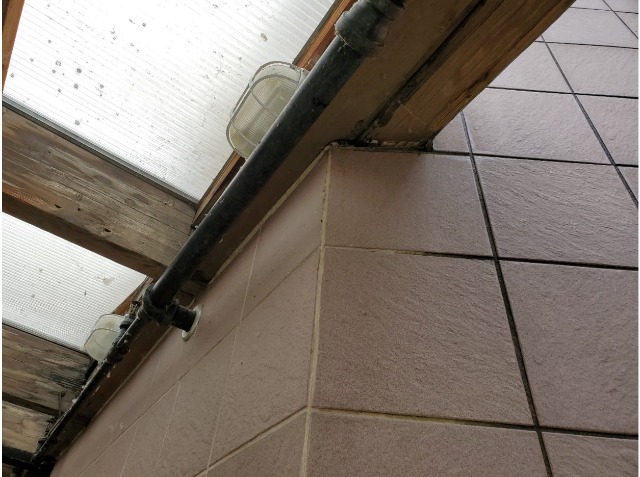
Intersection between front canopy beam and wall
