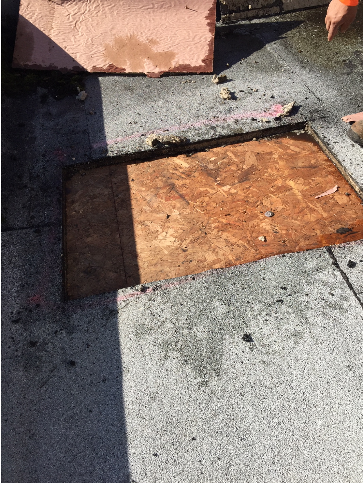
Typical observed condition of roof sheathing
