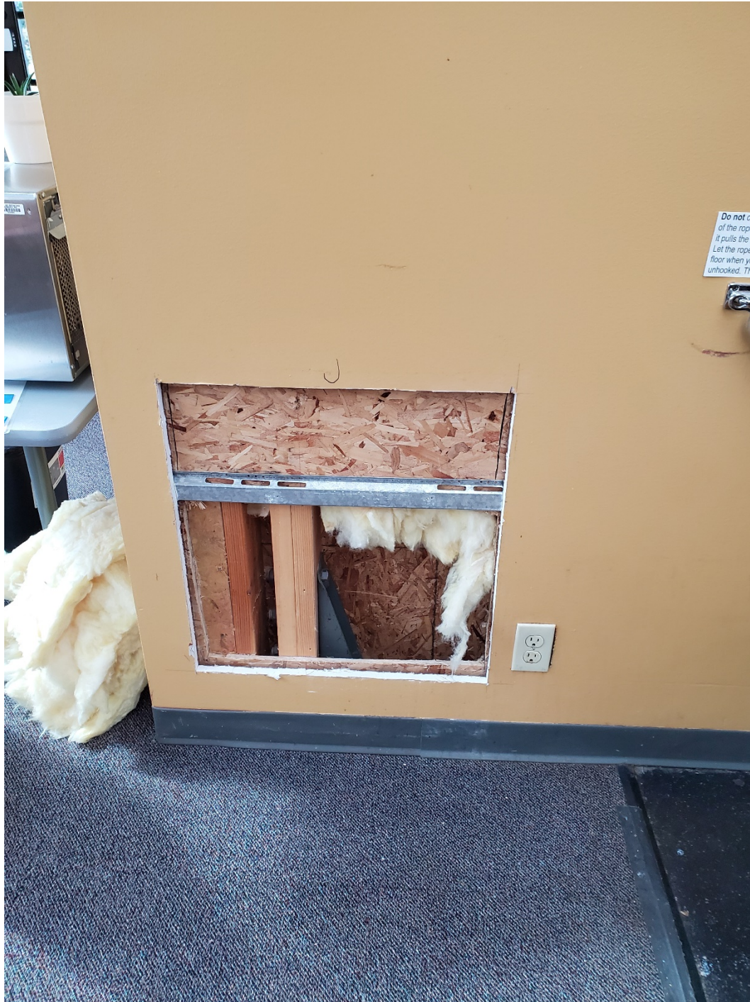
Typical observed condition of interior shear wall, including hold down
