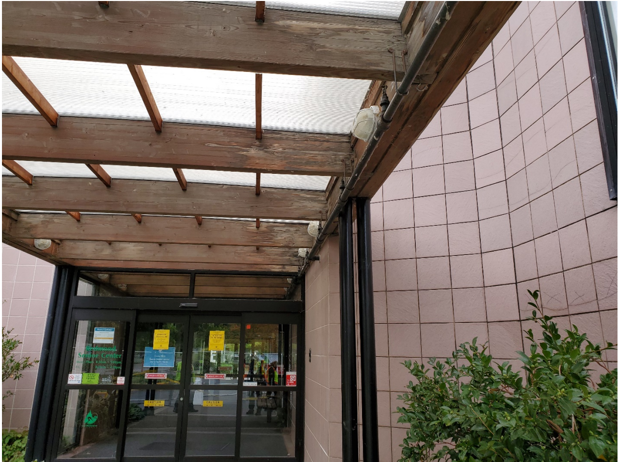
View of canopy cross beams
