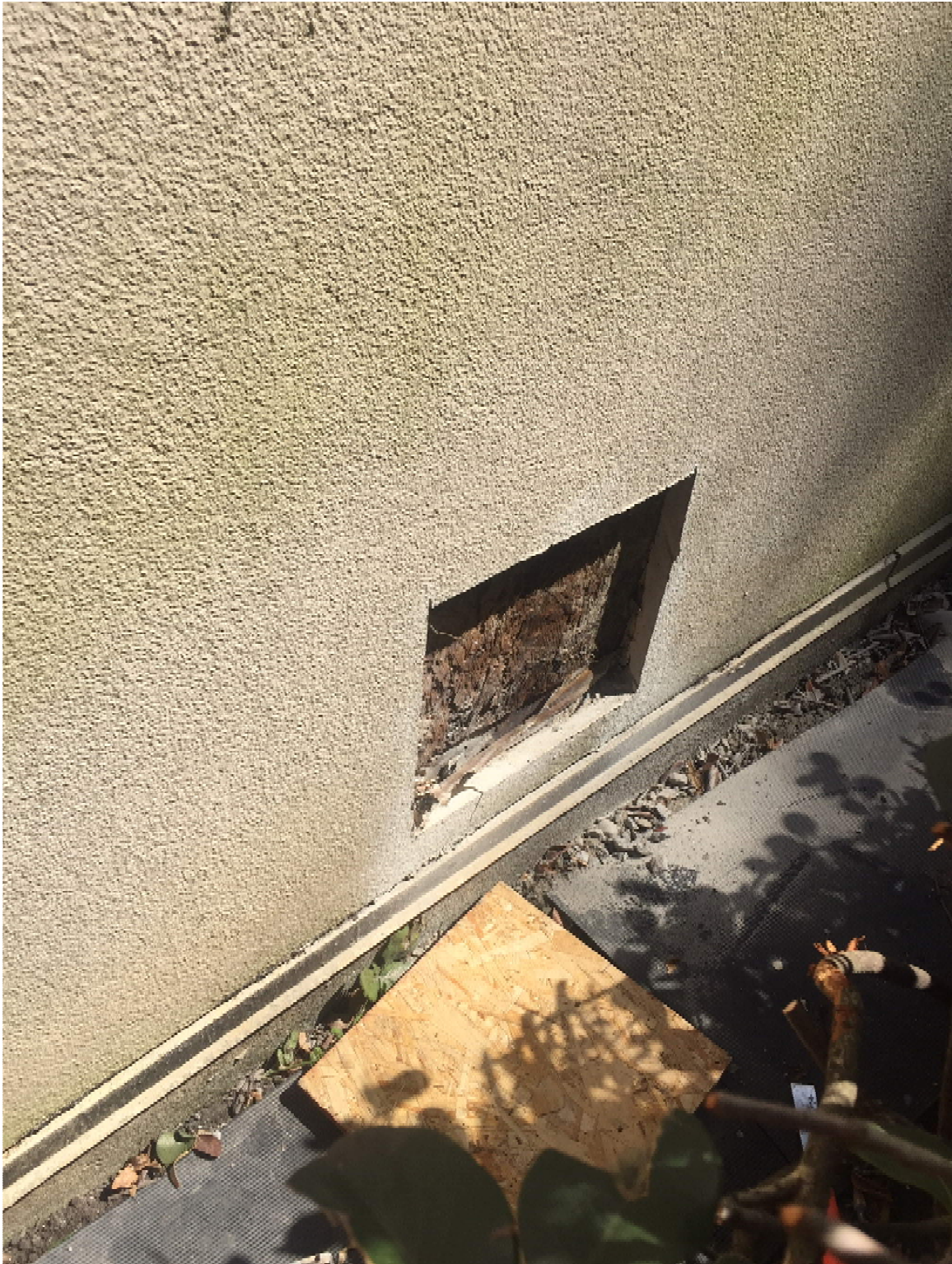
Figure 1 - Typical opening showing signs of significant deterioration of OSB sheathing.
