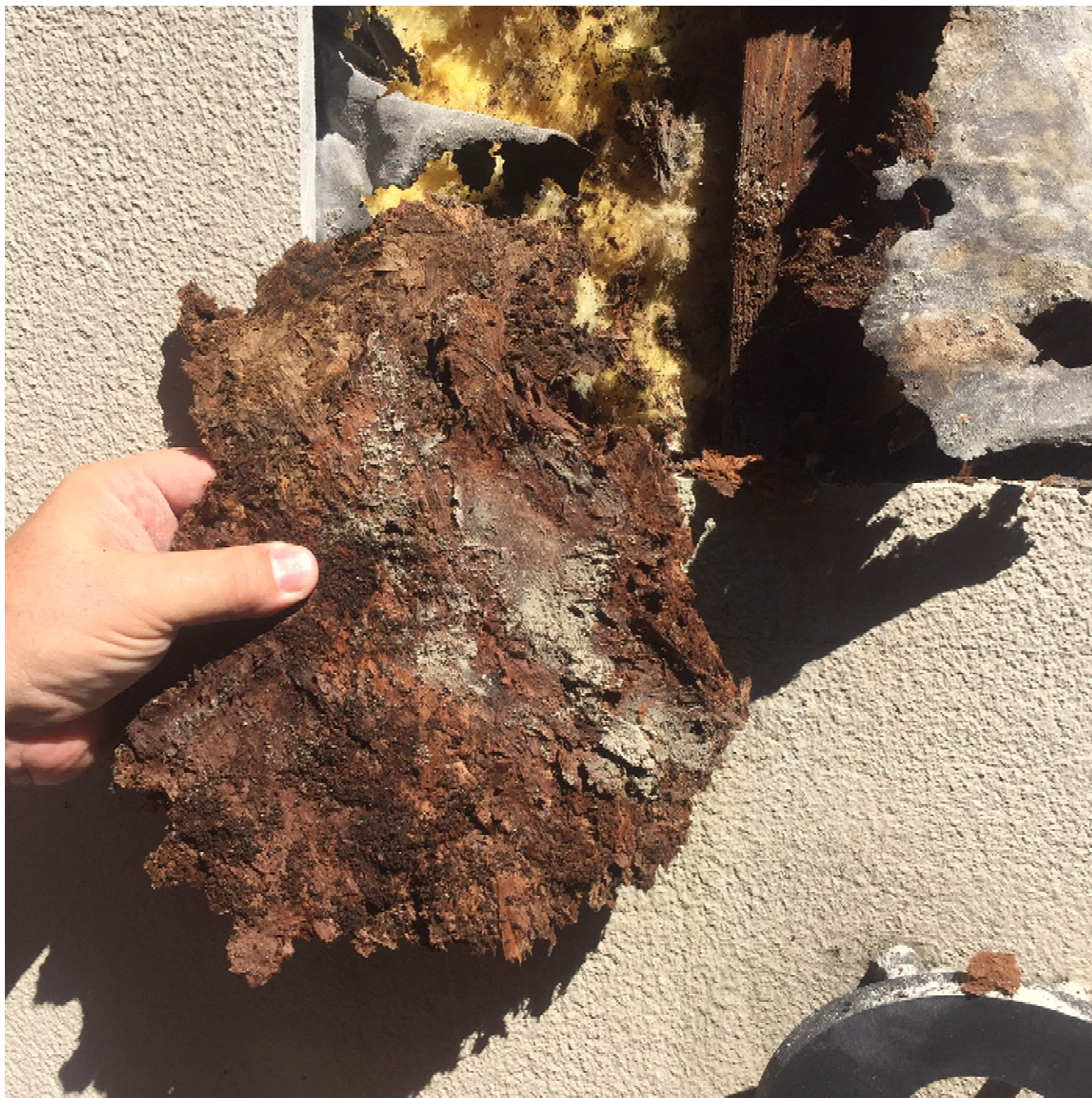
Figure 2 - Significant OSB sheathing deterioration.
