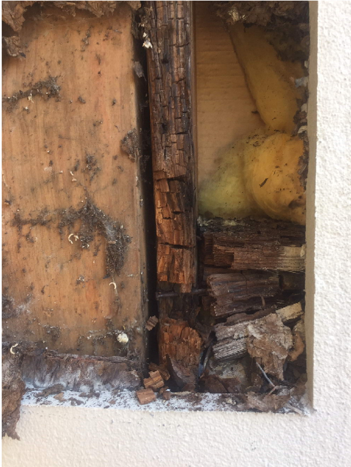
Figure 3 - Sample of significant deterioration in wood stud wall framing.
