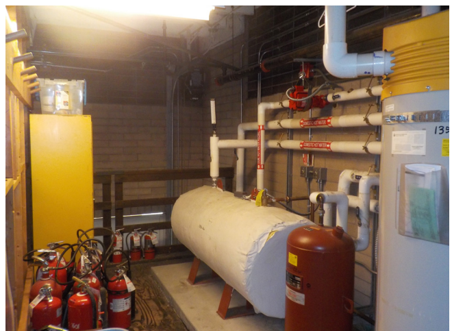
Figure 14. Mechanical equipment and supplies stored in a seismically vulnerable mezzanine at Fire Station 11
