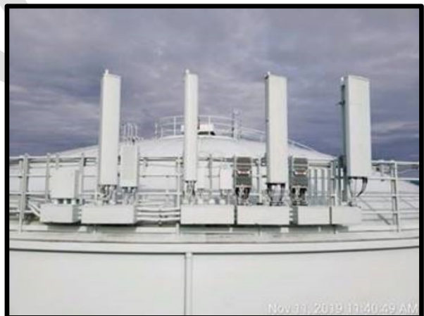
FIGURE 3 LEASED TELECOM EQUIPMENT MOUNTED ON TOP OF THE ROSE HILL WATER TANK
