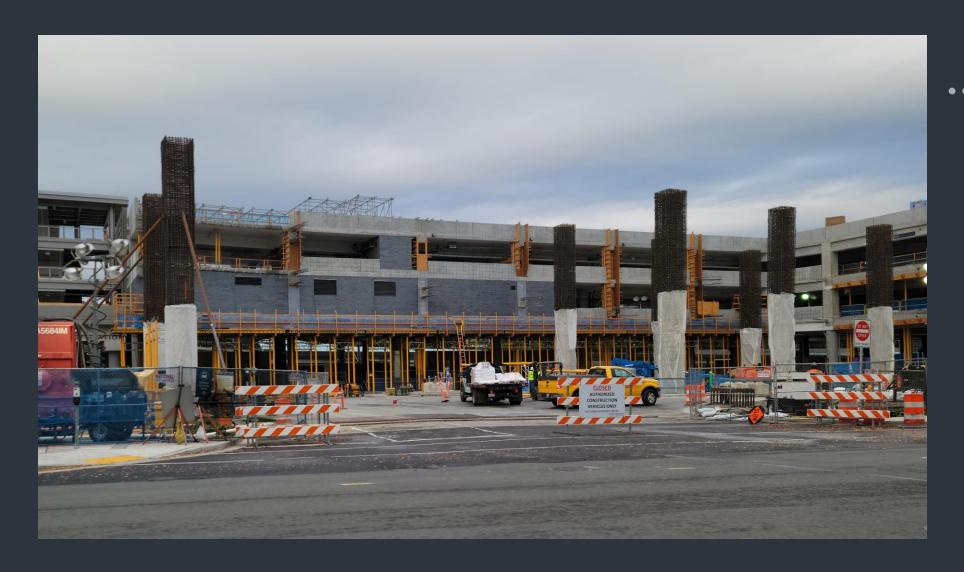
Columns for new ramp structure (replacing about 1/4 of structure)
