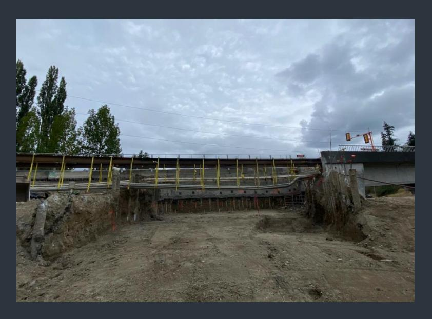
Excavation and soil nail walls with temporary signal to right
