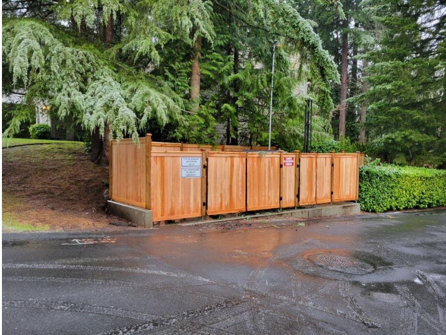
Wastewater Lift Station 15 after project completion
